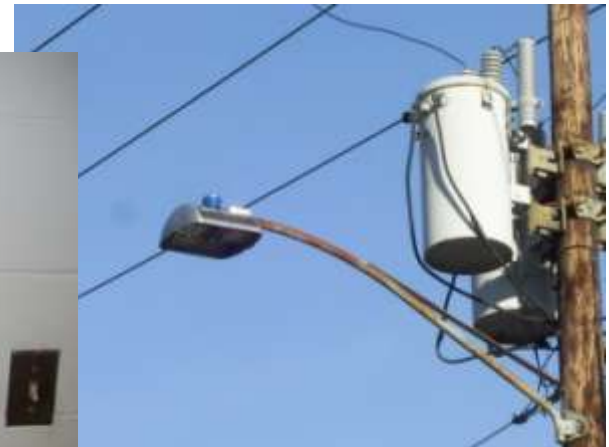
New 88w LED lamp and installed
