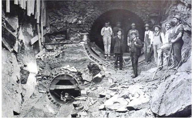
9.1. Just east of Austin Farm in Dorchester, Canterbury Brook was made to flow underground through the large conduit in the upper right, parallel to a smaller sewer line (lower left). *From Street Department Annual Report, 1906.*
