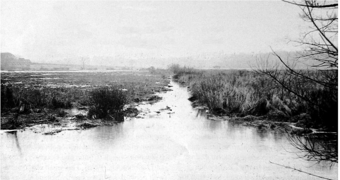
7.4. The BNC wetland as viewed from Morton Street around 1900. Note the straight culvert (recently created by Arthur Austin's workers) channeling water through the center of the wet meadow, as well as the absence of trees around the wetland—a very different place than it is today. *Photo from the Boston Water and Sewer Commission.*
