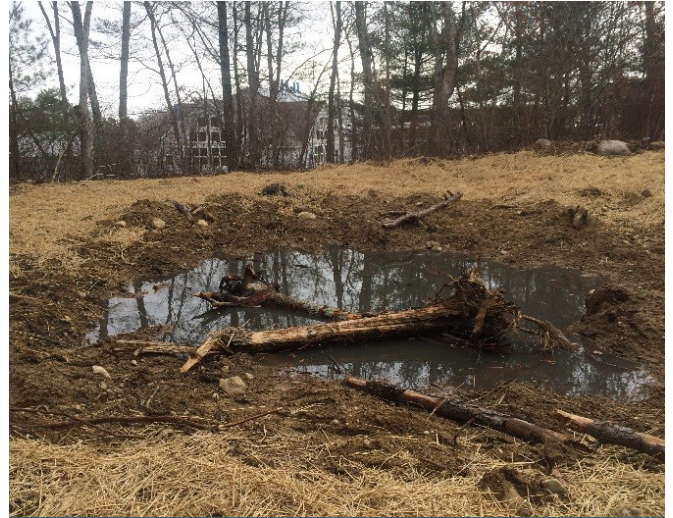
A liner wetland at Falmouth Academy in Falmouth filled with rainwater two weeks after creation.
