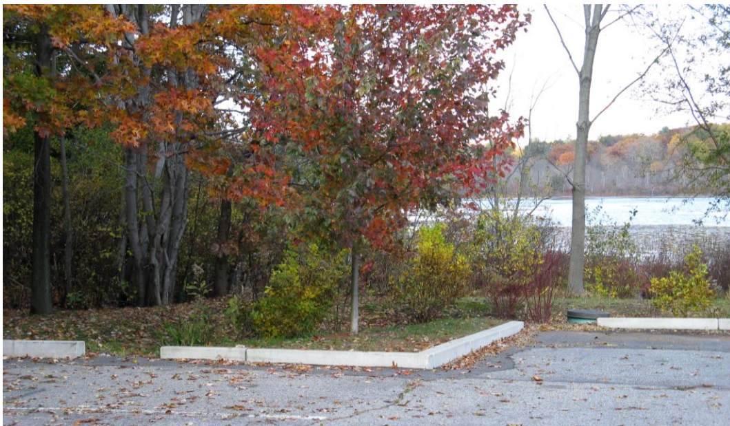
One of five bioretention areas at Hammond Pond
