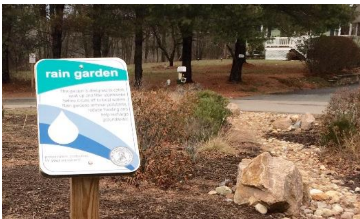
Anchorage Road rain garden
