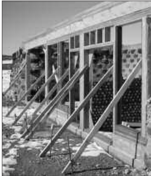
Earthship under construction
