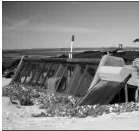
View of the south side of an Earthship
