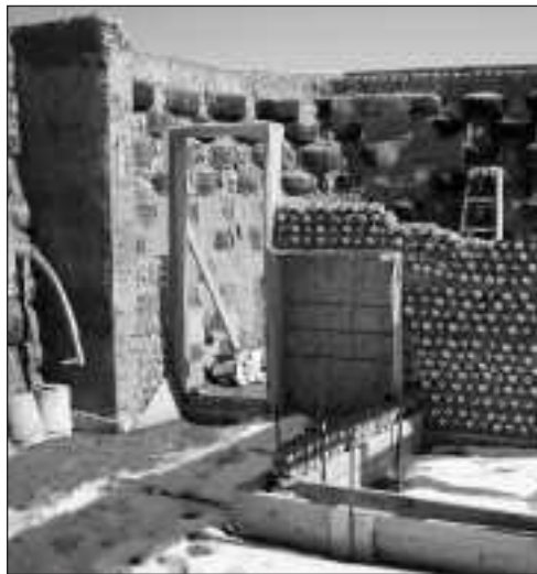
Walls are constructed with used tires and recycled aluminum cans.
