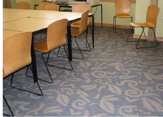
Carpet tiles contain 54% recycled content and contribute to a healthier indoor environment by emitting only low levels of Volatile Organic Compounds (VOCs).
